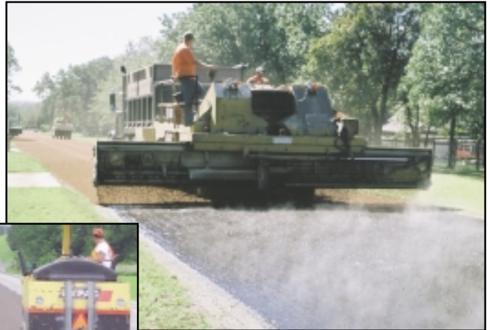
(Above) ASTM # 8 LWA applied at 115 SY/CY over CRS-2S at 0.40 GAL/SY in a county residential street • (Left) Pneumatic rubber-tire roller
