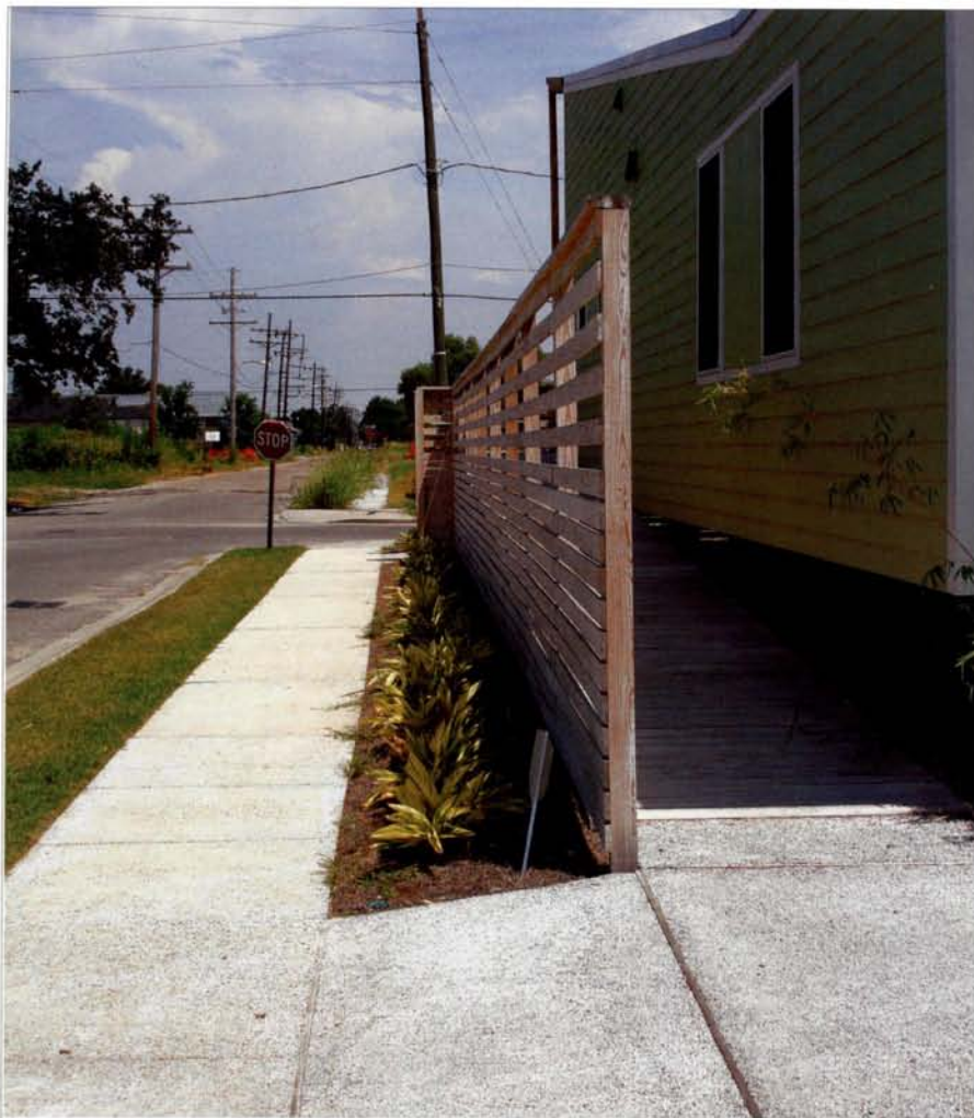
Pervious concrete has been used in lieu of conventional flatwork for a post-Katrina New Orleans neighborhood.
