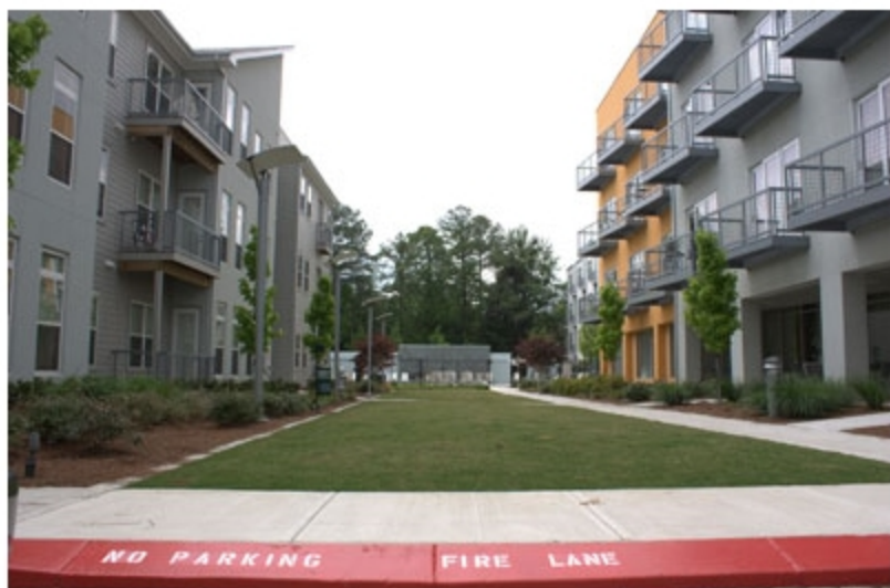
The fire lane offers storm water and green space benefits.
